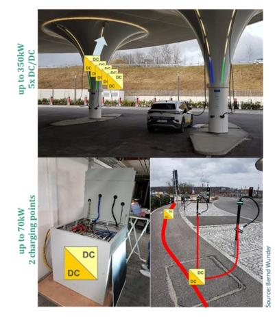
➡ Without galvanic isolation between the charging points, this topology is normatively not authorized (IEC 61851-23 ED2 FDIS 2022)
